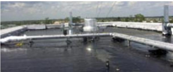
An emergency roof (shown) was installed after Hurricane Charley blew the mechanically attached PVC membrane roof covering off the concrete deck of the Fawcett Memorial Hospital.
