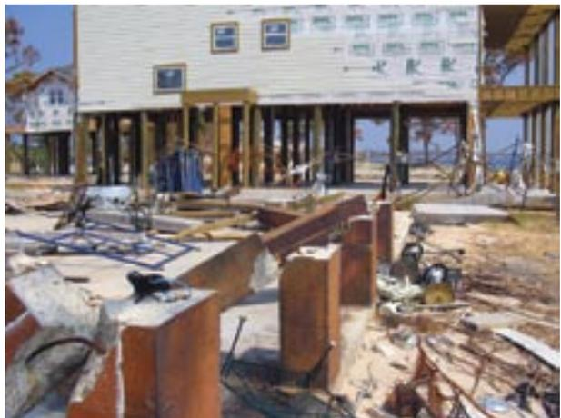
High flood levels during Hurricane Ivan and lack of structural capacity to withstand waves and debris loads caused this reinforced pier foundation to fail.
