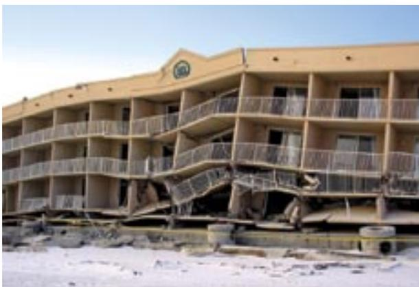
A multi-family condominium collapsed after Hurricane Ivan due to erosion of supporting soil under the shallow foundation.
