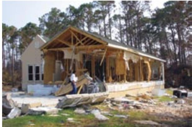
Flood water from Hurricane Ivan exceeded the required elevation of the top of the lowest floor supported by the stem wall foundation for this house leading to severe damage caused by waves and debris impact.
