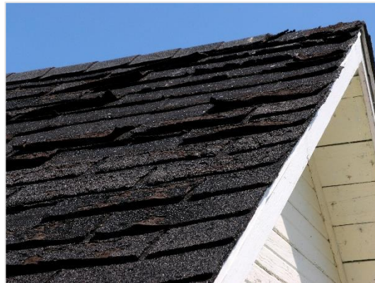
Loose/Brittle Shingles
