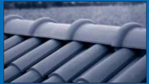
Clay or concrete tile is becoming more and more popular as a roof covering. But loose tile can become windborne missiles in hurricane-force winds if they are not installed properly.
