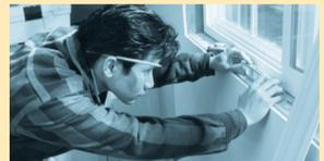
Impact-resistant windows and doors, and impact-resistant coverings must be installed according to the manufacturer's instructions to ensure effective protection of your home's openings. Read the installation instructions that accompany the product you have chosen for installation. You may choose to hire an inspector to confirm the proper installation of your opening protection products prior to making full payment to the installer.
