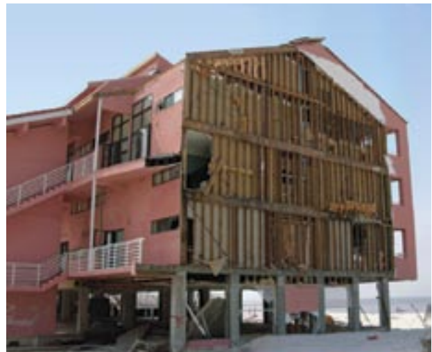
Example of wall cladding failure. The building had synthetic stucco installed over molded, expanded polystyrene insulation and gypsum board. The gypsum board blew off during Hurricane Ivan.
