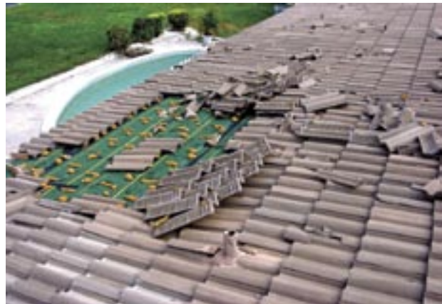
In addition to the damage shown in this photo, this one-story roof lost virtually all of the hip and ridge tiles during Hurricane Charley. (Punta Gorda Isles)
