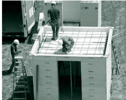
constructed in accordance with the prescriptive designs of the FEMA 320 Publication, *Taking Shelter From the Storm: Building a Safe Room Inside Your House*. Deviations from FEMA 320 and manufactured safe rooms must be tested at an approved laboratory such as the Wind Science and Engineering Research Center at Texas Tech University.
