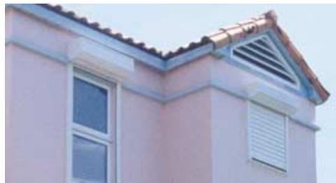
use above the ground floor, electric roll-down shutters can be operated with the flip of a switch inside the home.
